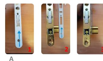
After fitting the lock body in the door thickness, remove the frontal plate and screw the cylinder using the screw supplied.
