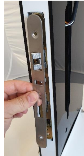
3. Fit in the front plate.
