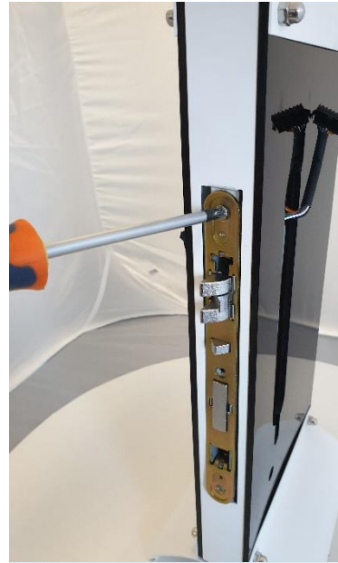
2. Fit in the lock and set in place using the fixing screws.
